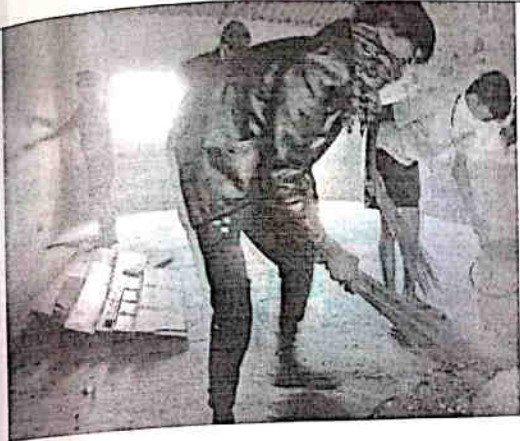
Cleaning of ZP School building (Before)
